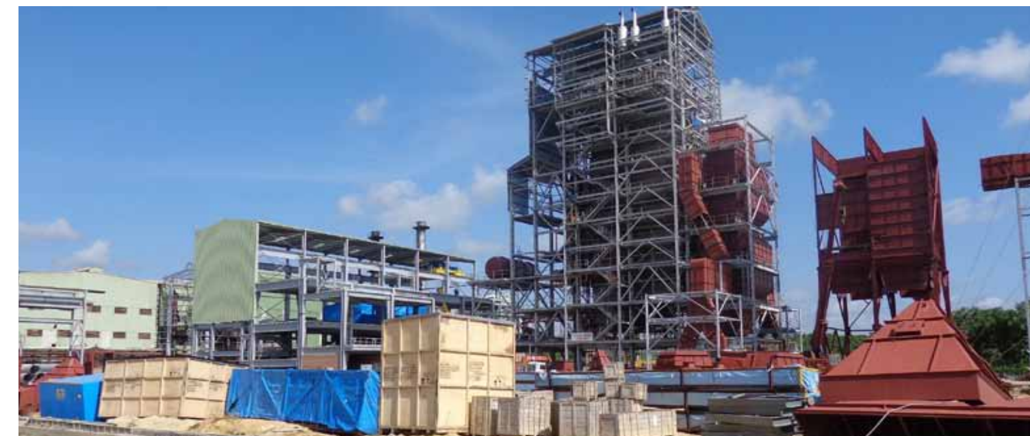
New Boiler & Turbine House under erection for Season 2015 - 2016
