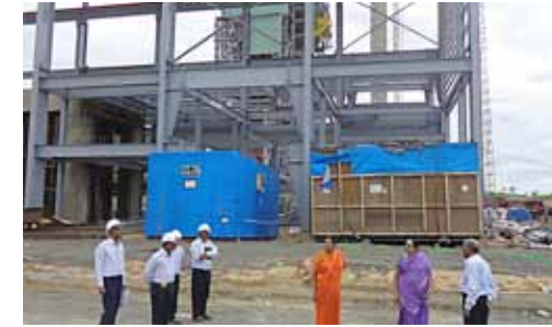
STG Building & Boiler Erection Site
