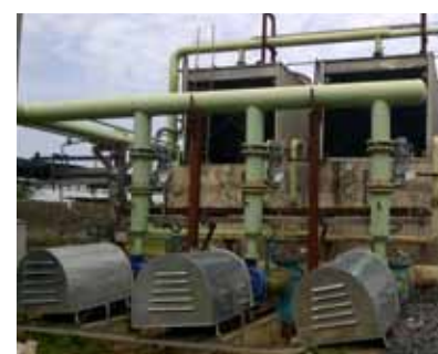
To improve the capacity of Raw Mill, the central feed pipe size was reduced and 2 hoppers were installed at the inlet of hot air chute to remove unground material. New multi stage pumps were installed in place of old pumps to increase flow rate and water injection nozzles were replaced with high efficiency nozzles.
