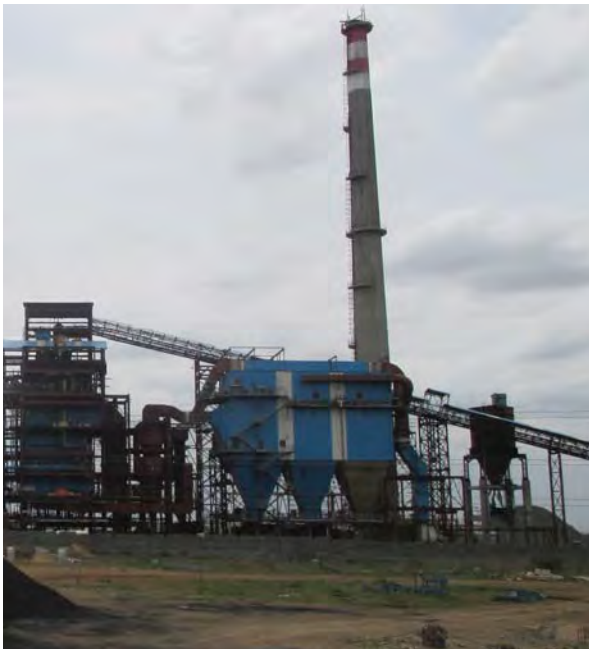
Captive Power Plant - Muktyala
