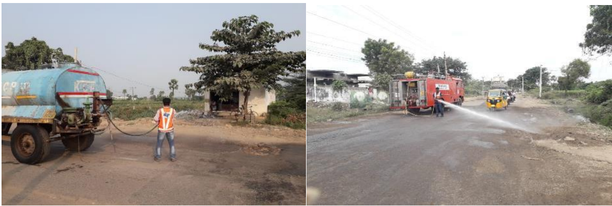
Water spraying in K. Agraharam village Main Road
